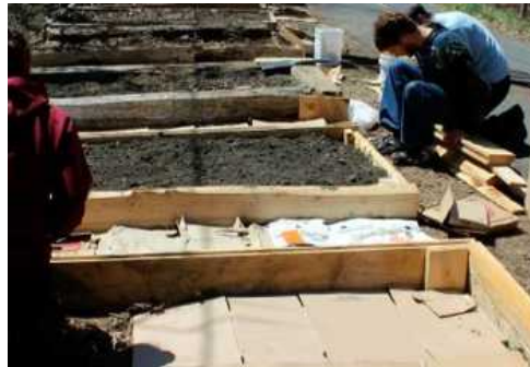
Putting in raised veggie beds on the Rail Trail
